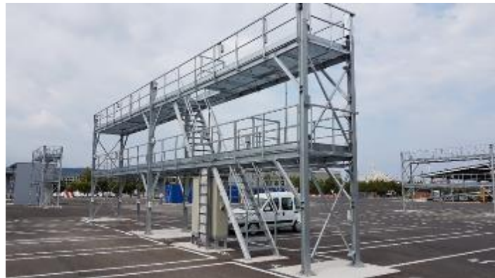
Gallery with power supply for refrigerated containers
